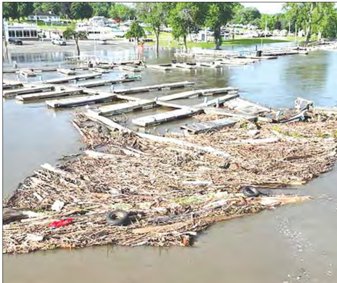
Floating debris from collapsing docks.
