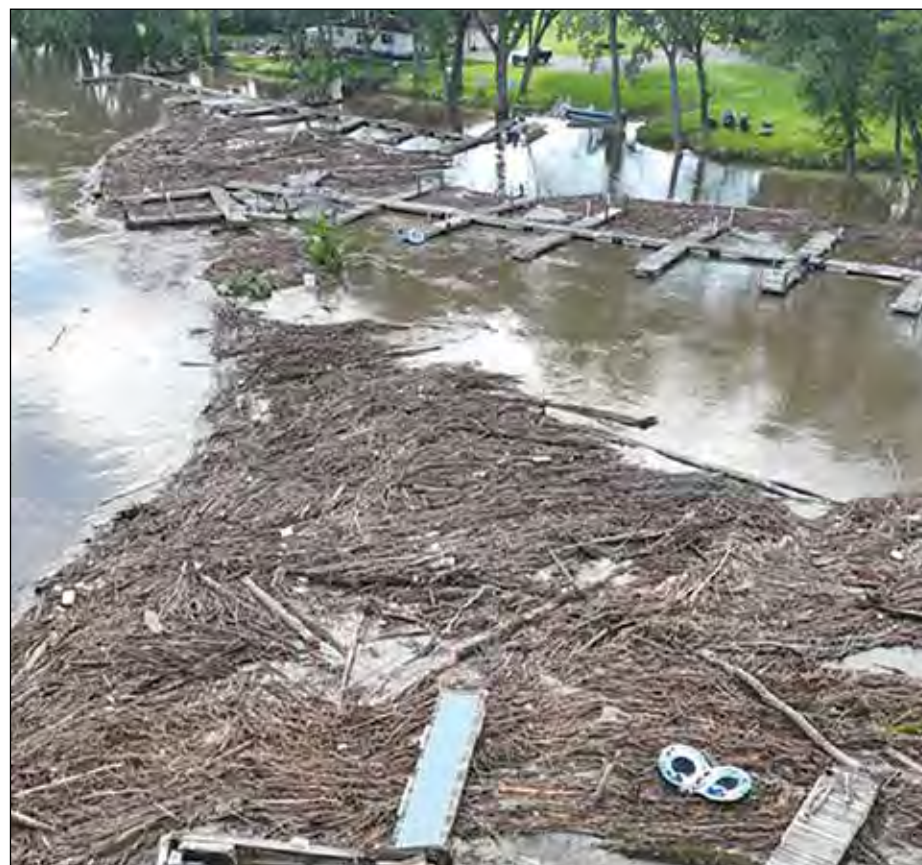
Debris cluster from collapsing docks.
