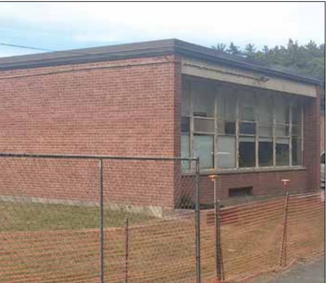
Tech installations will be starting soon on the project.
